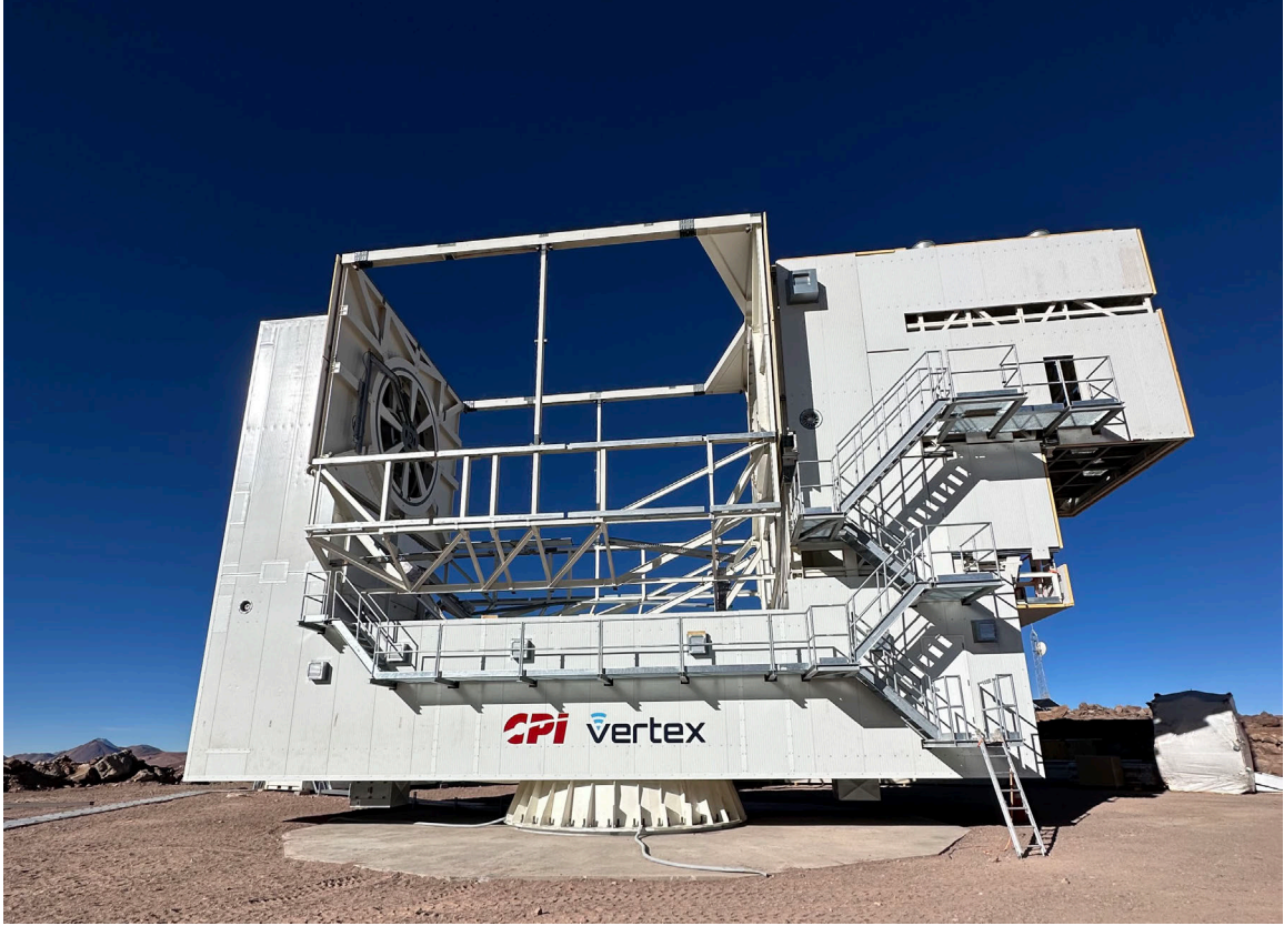
Figure 11. The Simons Observatory Large Aperture Telescope. Not pictured are the primary and secondary mirrors, which are due to be installed in early 2024.
