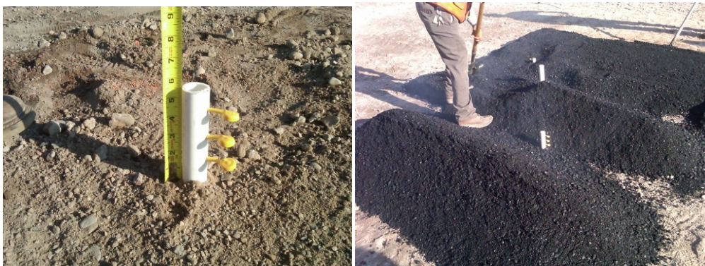
Figure 7 – Pavement Temperature Sensors Installation
