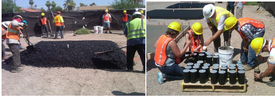
Figure 6 – Construction of Porous HMA and Sampling of PCC Materials
