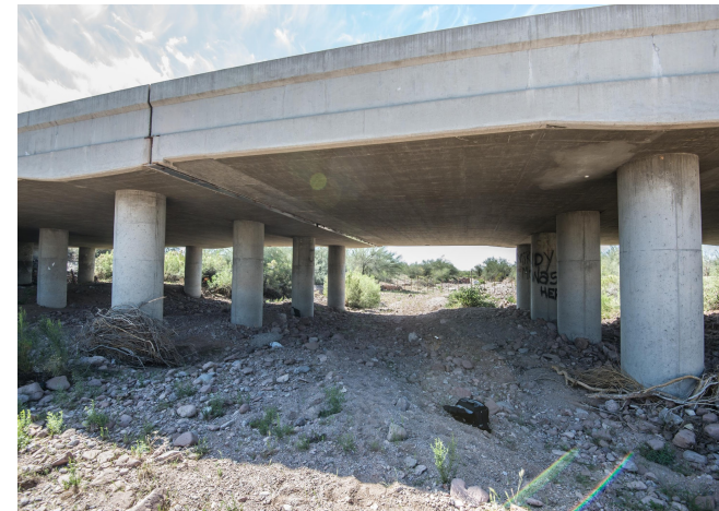
Figure 4-11: Siphon Draw Overpass Before
