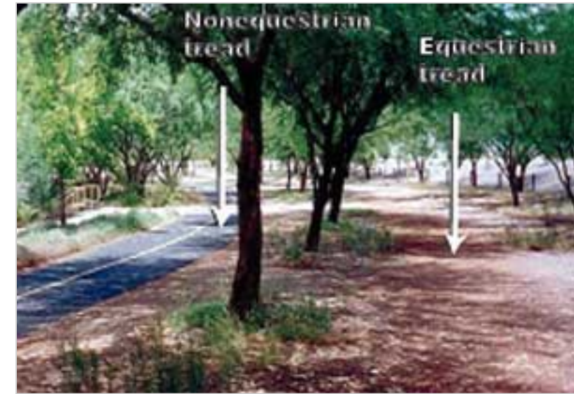
Figure 2-6: Example Multi-use Trail with recommended surface material (AmericanTrails.org)
