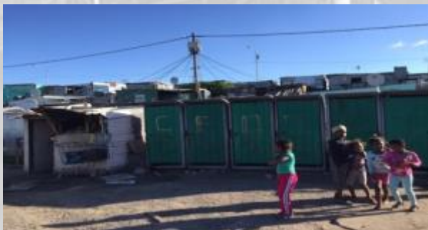
Image 1.6: Existing Restroom Facilities
