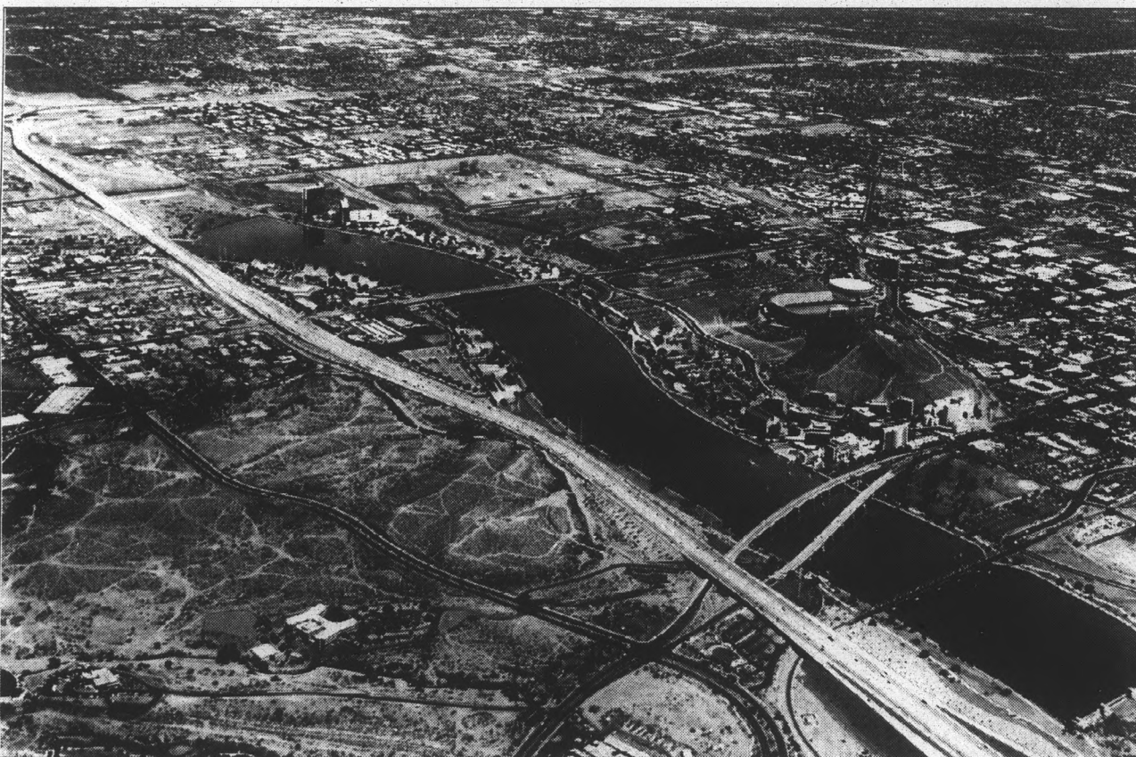
An artist's depiction of the Rio Salado Town Lake shows what the area will look like once completed.
