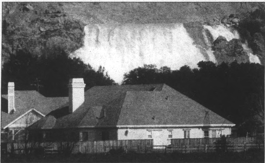
A home sits safely in the foreground of the Anderson Reservoir dam spillway Monday in Morgan Hill, Calif. Water officials said 2,800 cubic feet per second of water is going over the spillway after recent heavy rains in Santa Clara County.
