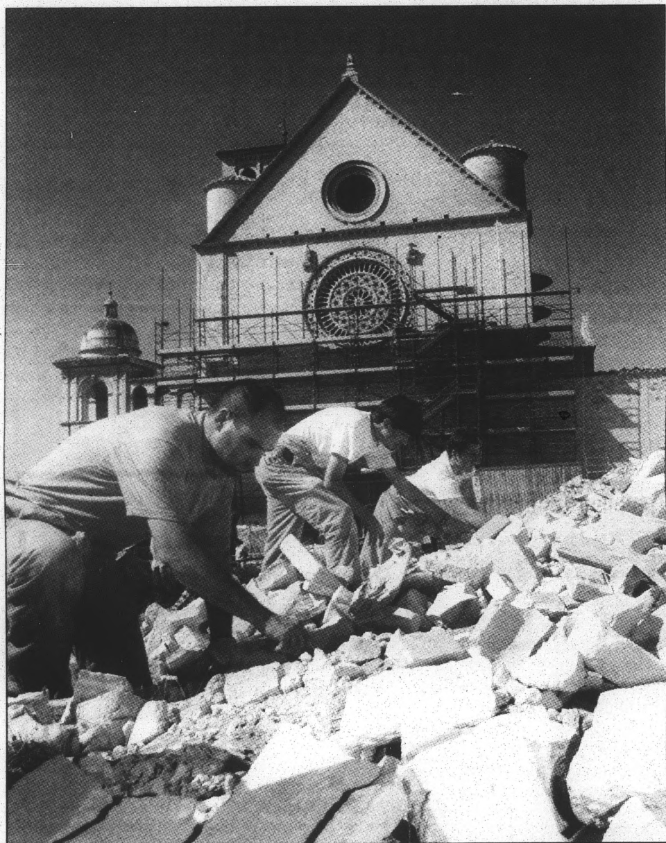
Volunteers search for pieces of frescoes amid the debris from the collapsed vault of the St. Francis Basilica of Assisi, background, Saturday. The vault, painted by Giotto and Cimabue, collapsed early Friday when a major earthquake struck central Italy. The scaffoldings on the Basilica facade were installed before the quake as part of an ongoing restoration effort.
