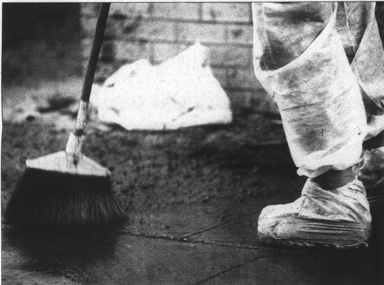
Lori Cain/State Press Protected from head to toe, workers contracted from Facilities Planning and Construction remove insulation from the roof of McClintock Hall Thursday afternoon. The protective gear is worn to prevent the fiberglass within the insulation from irritating the lungs, eyes and skin of the workers.
