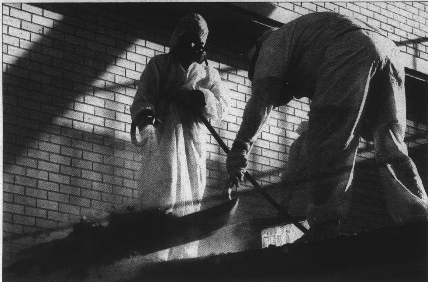
Lori Cain/State Press Protected from head to toe, workers contracted from Facilities Planning and Construction remove insulation from the roof of McClintock Hall Thursday afternoon. The protective gear is worn to prevent the fiberglass within the insulation from irritating the lungs, eyes and skin of the workers.
