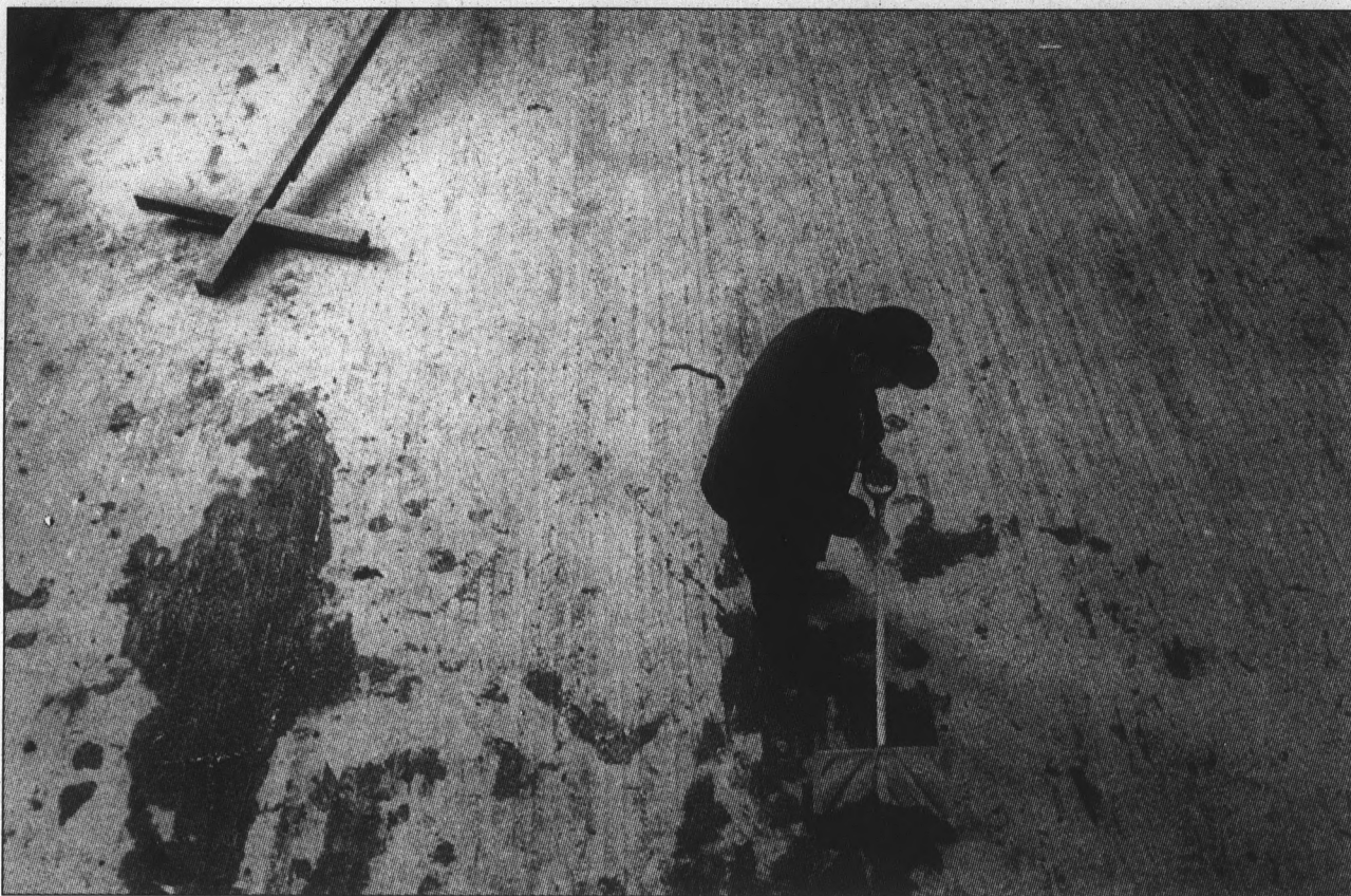
With an Easter cross lying on the floor behind him, George Lach uses a snow shovel to lift remaining wet mud from the sanctuary floor of the United Methodist Church in Falmouth, Ky., Sunday morning. The church, built in 1854, was unable to hold services Sunday because of the destruction caused by last weekend's flooding of the Licking River.
