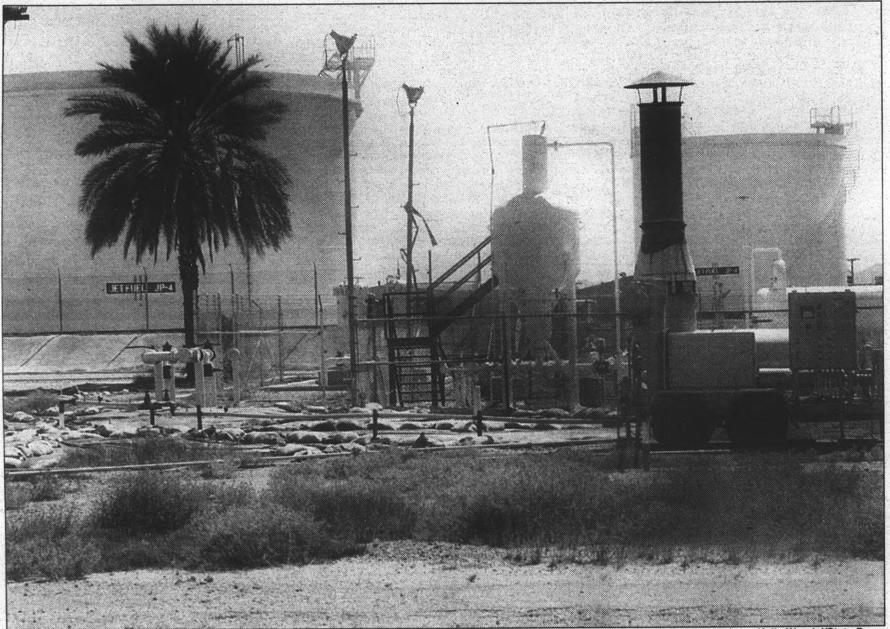
A soil vapor extractor is helping clean up a toxic waste site at ASU's new east valley campus.
