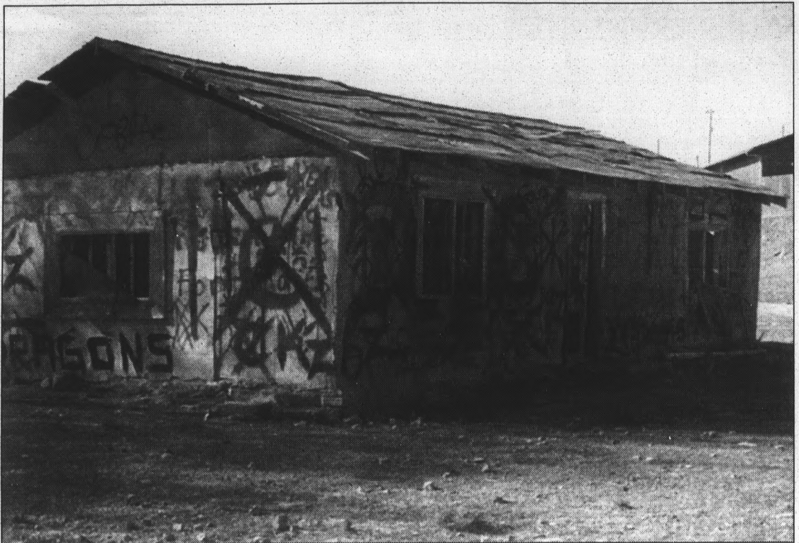
The scourge of urban America, spray-painted insignia of gangs, litters this building in Fort Defiance, Ariz. More than 200 miles from the nearest big city, gangs are being blamed for increasing beatings, stabbings and killings in the Navajo Nation.
