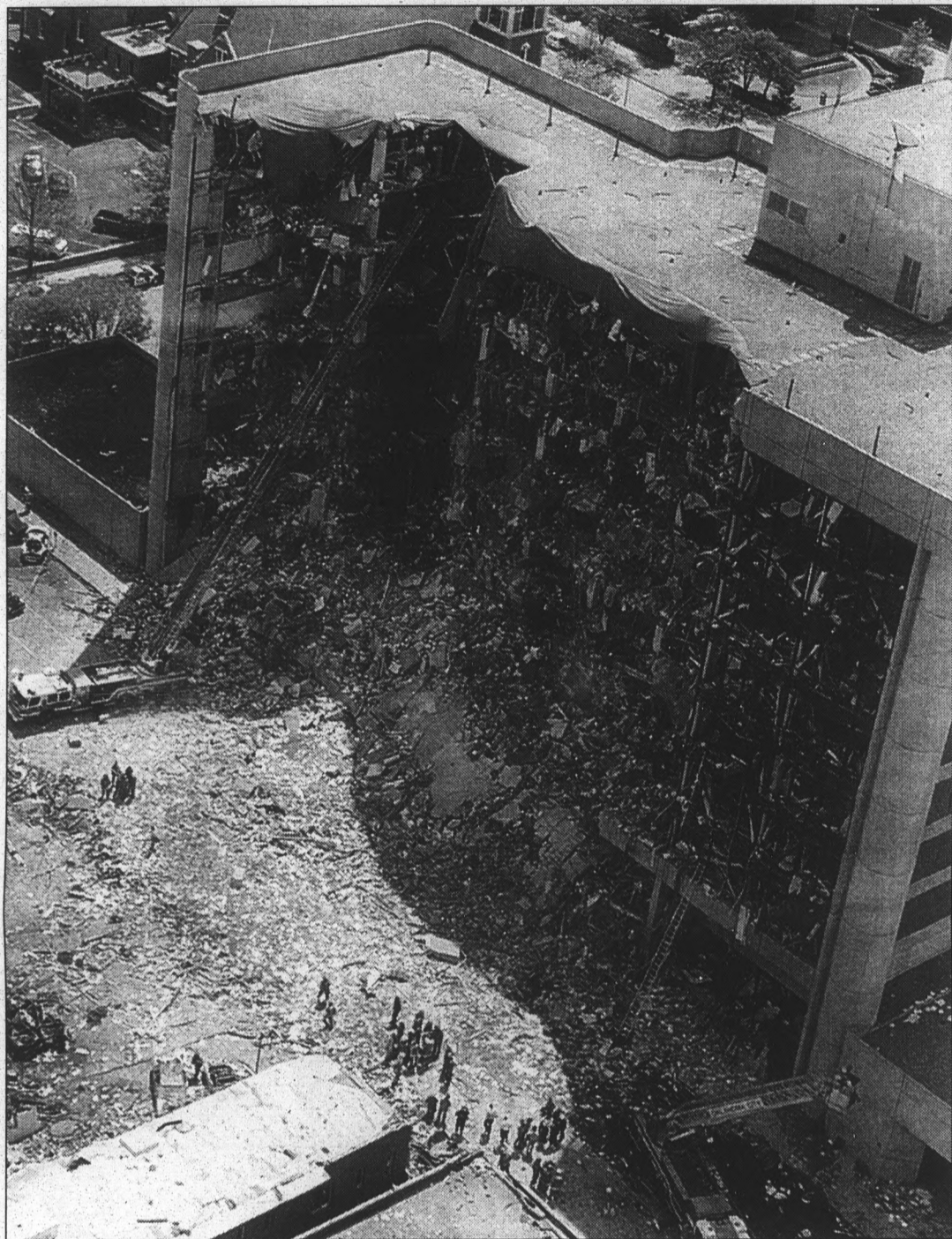
The Alfred Murrah Federal Building in downtown Oklahoma City sits in ruin after a car bomb tore the structure in half shortly after 9 a.m. Wednesday. At least 31 people died in the blast, with at least 200 injured and 300 still unaccounted for. See related stories, pages 3 and 7.
