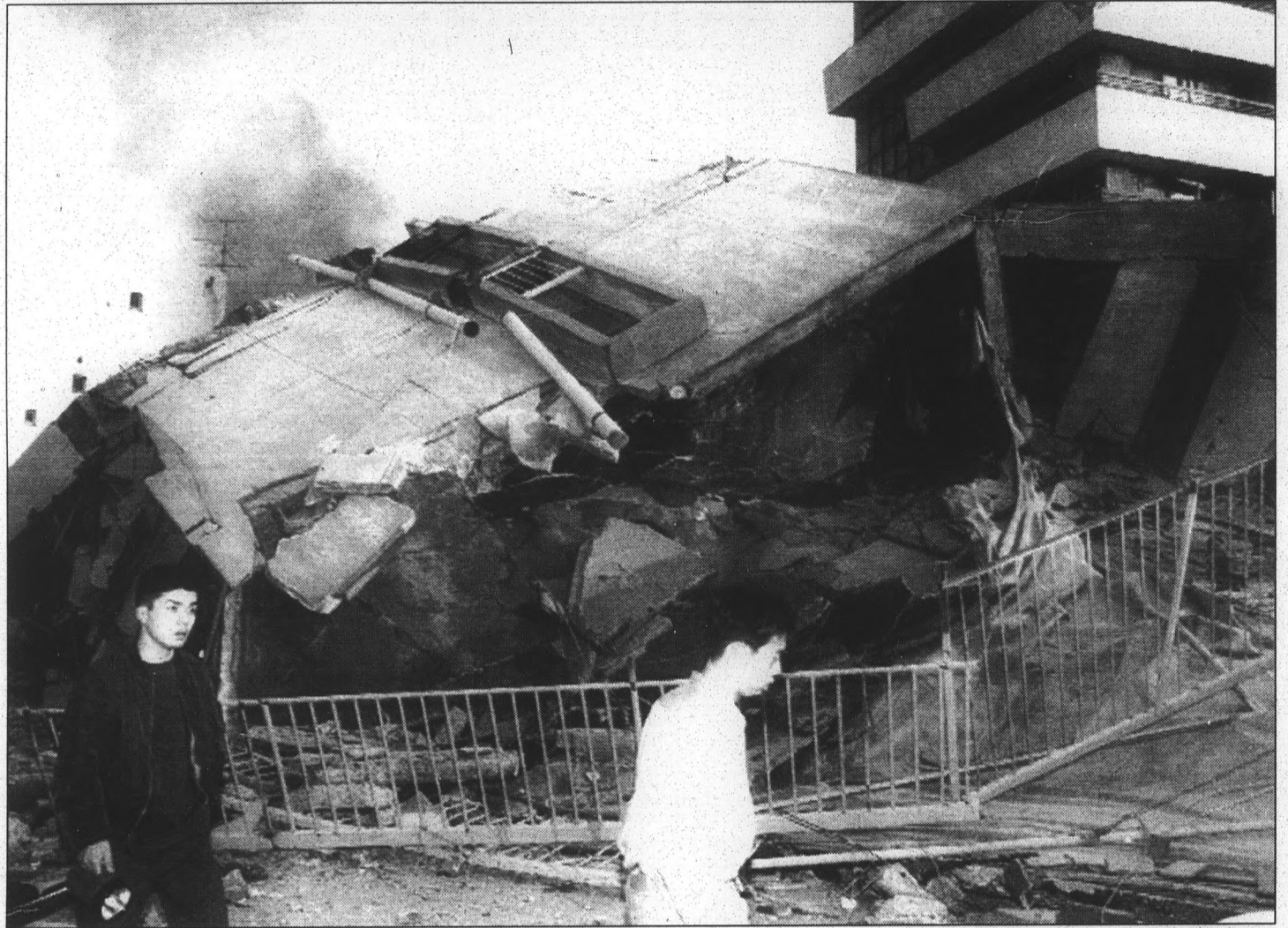
People walk past a collapsed seven-story apartment building in Nishinomiya, Japan Tuesday. Tuesday's 7.2 earthquake in western Japan left 1,800 people dead and more than 6,000 injured.
