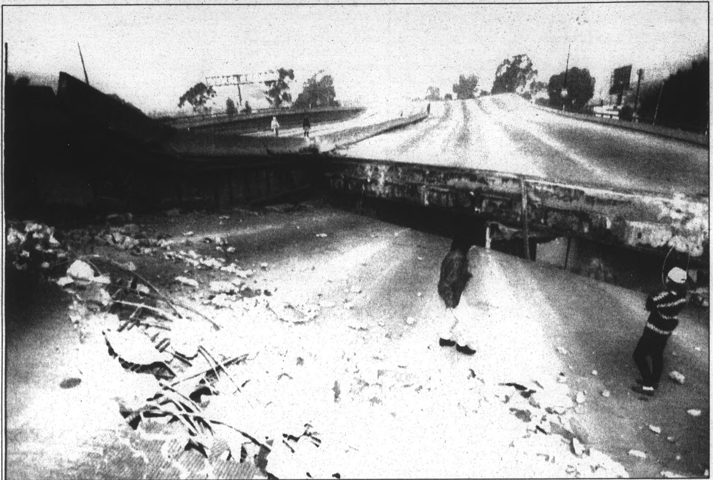
The Santa Monica freeway is split apart near the La Cienega overpass early Monday morning after a major quake struck the Los Angeles basin shortly before dawn.
