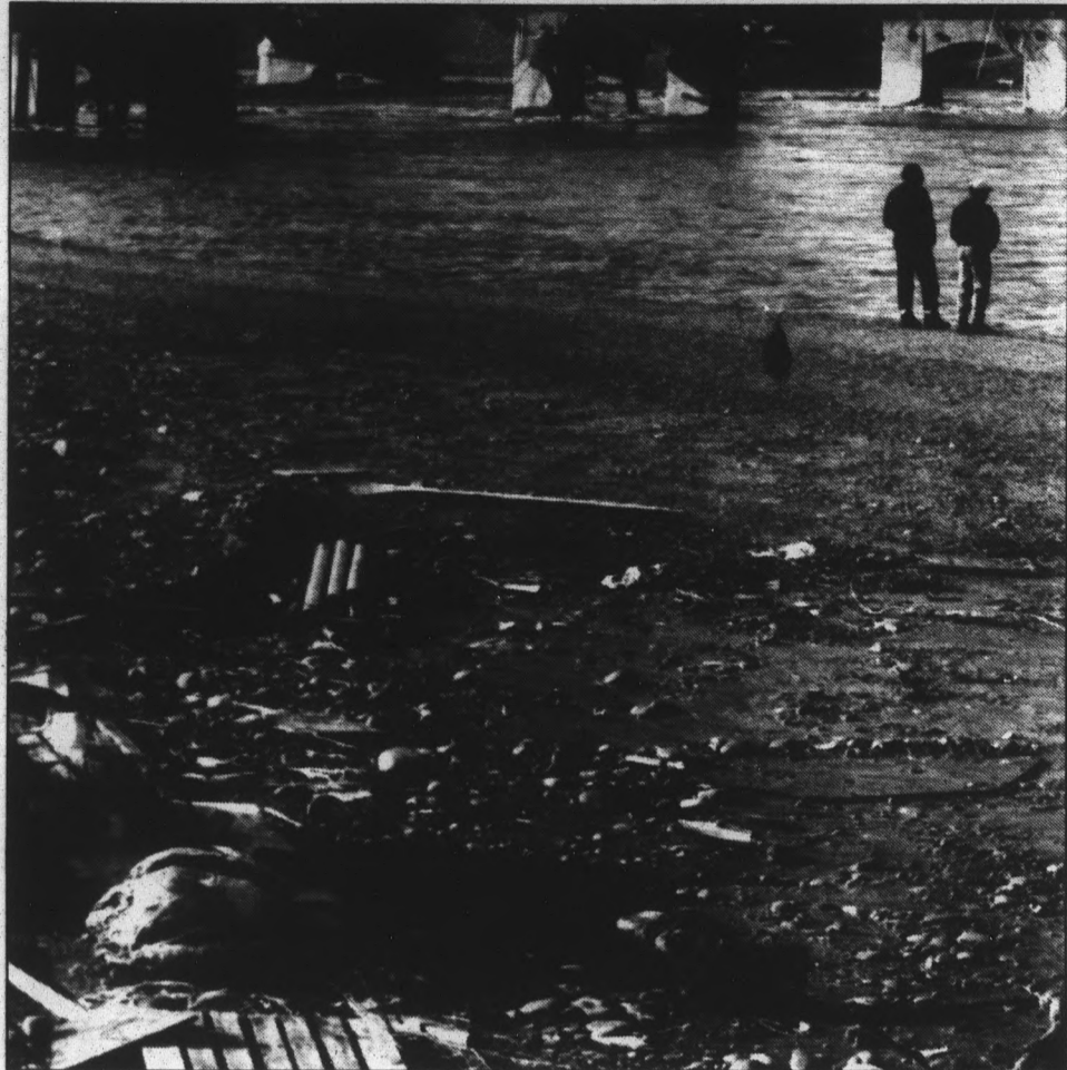
Two men survey the damage to the Mill Avenue Bridge by the raging floodwaters of the Salt River. Darryl Webb/State Press
