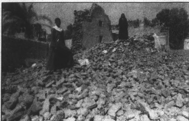
Two residents of the town of Roda, near the epicenter of Monday's earthquake, stand in front of the remains of their house Tuesday. Officials blamed many of the more than 400 deaths on old, weak buildings and poorly constructed new ones.
