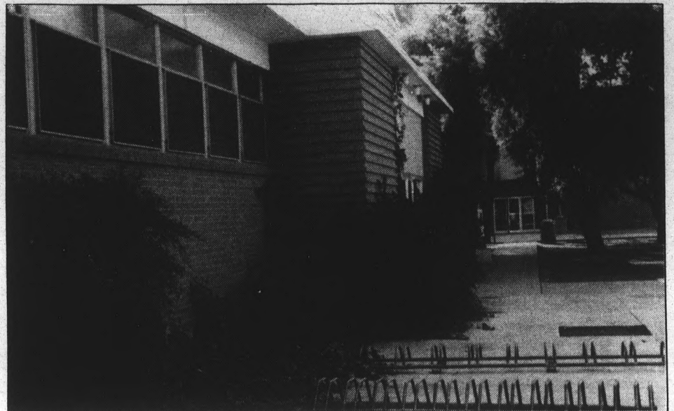
ASU is currently planning the demolition of the campus racquetball courts and the swimming pool along Orange Street to make way for the construction of the new Computer Network Services building.
