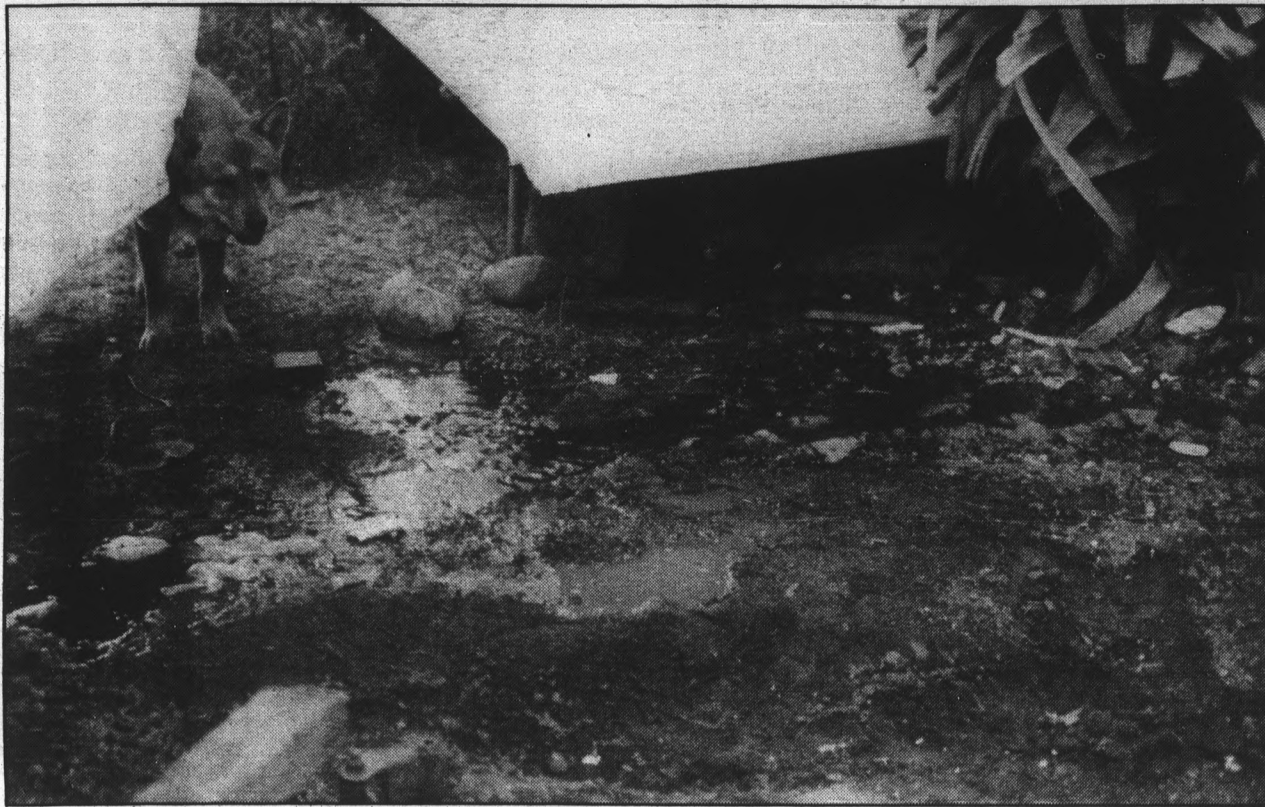
A pool of raw sewage accumulates in the Apache Trailer Park in this photo, taken in 1989.
