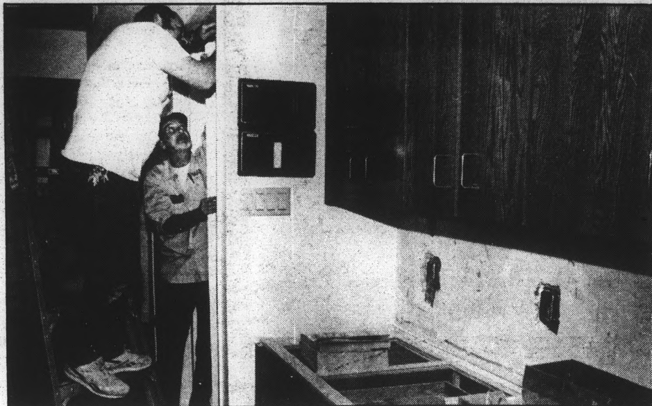
Bill Kerns helps Leonard Quenneville (on ladder), install a doorjamb in the main kitchen area in the University House. Quenneville, who works at the Physical Plant, helped renovate the house four years ago.
