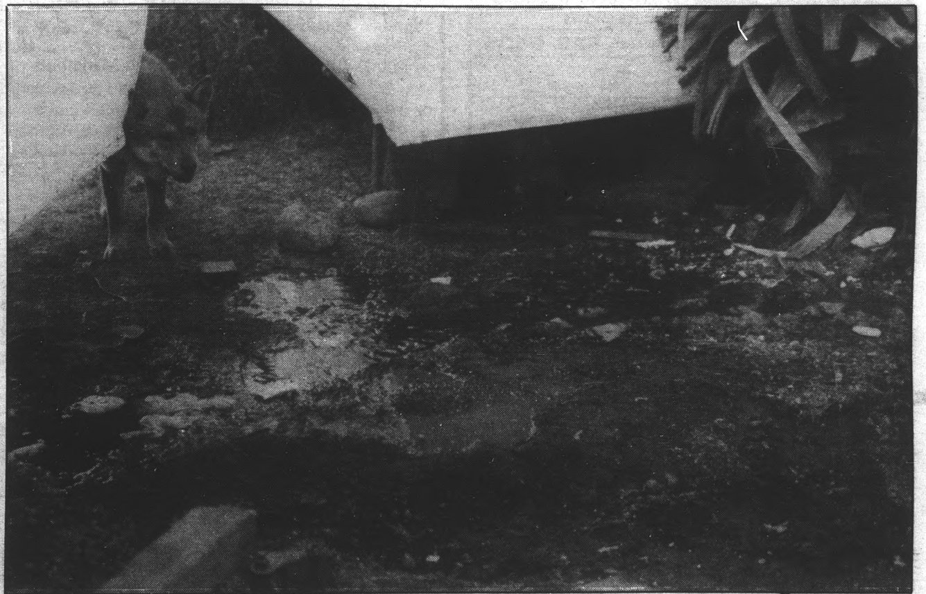
Raw sewage seeps between two mobile homes at Apache Trailer Park, 735 W. Apache. ASU, which owns the park, is suing three residents who say they will not pay their rent until the sewer system is replaced.
