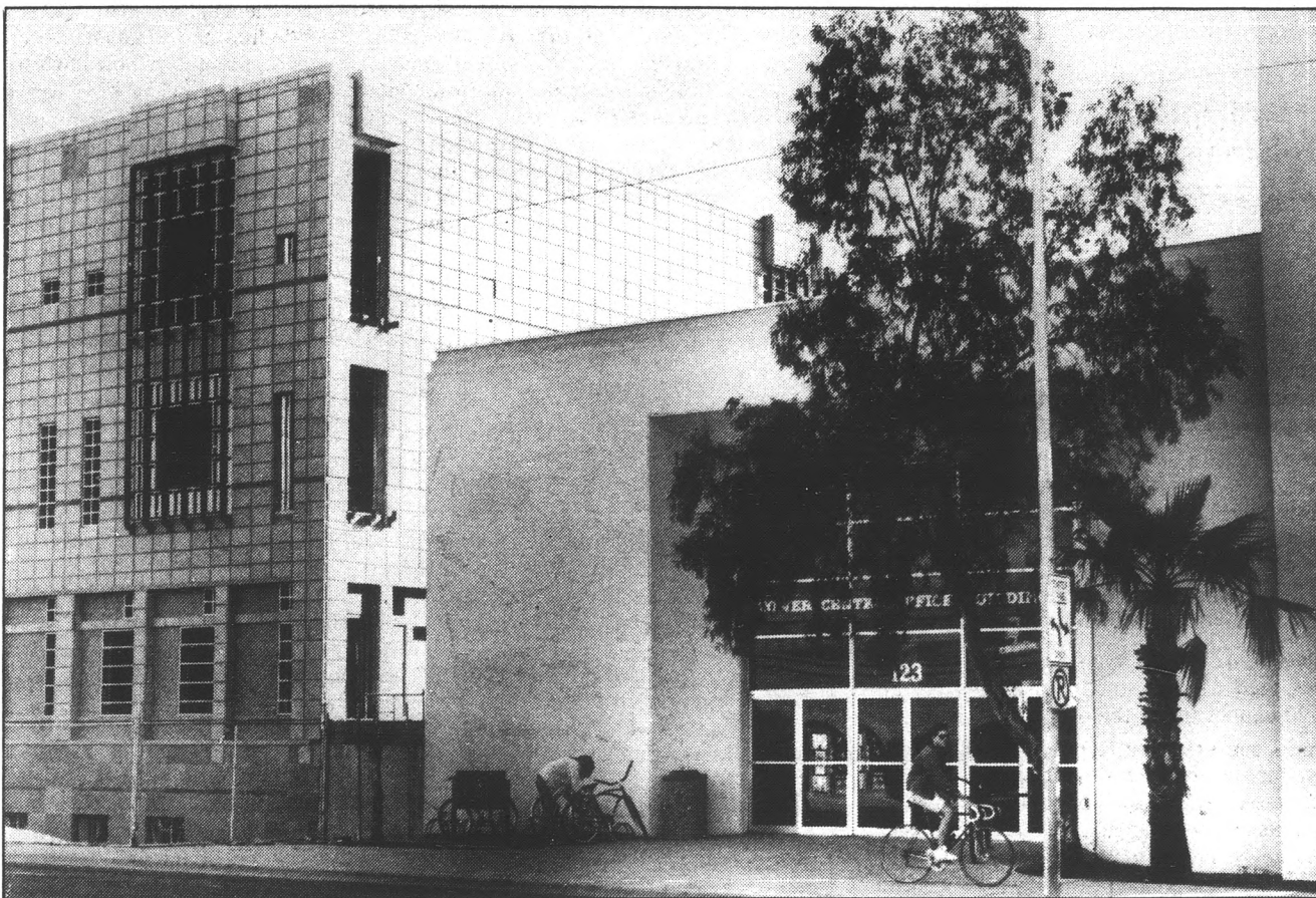
Tower Center (right) currently houses the KASR studios. Although an official date has not been set, the building will probably be torn down sometime after the completion of the Architecture Annex (left). KASR adviser Fredric Leigh would like to move the station to Stauffer Hall, but there is no space available.
