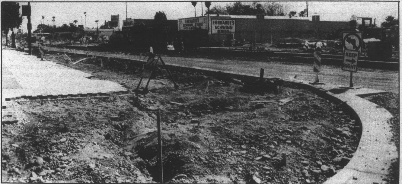
The Southeast corner of Mill Avenue during the $2.3 million construction project.
