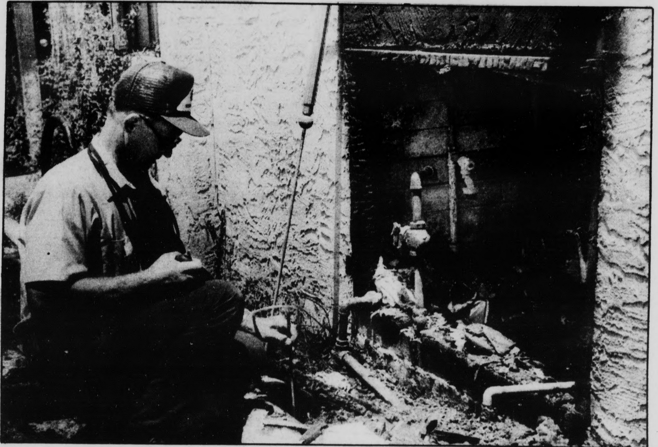
L. Al Nilsson, a service technician for Southwestern Gas, uses a gas scope to check for underground leaks at the Campus Inn Apts. A fiery ignition there Friday seriously injured manager Archie Stone.
