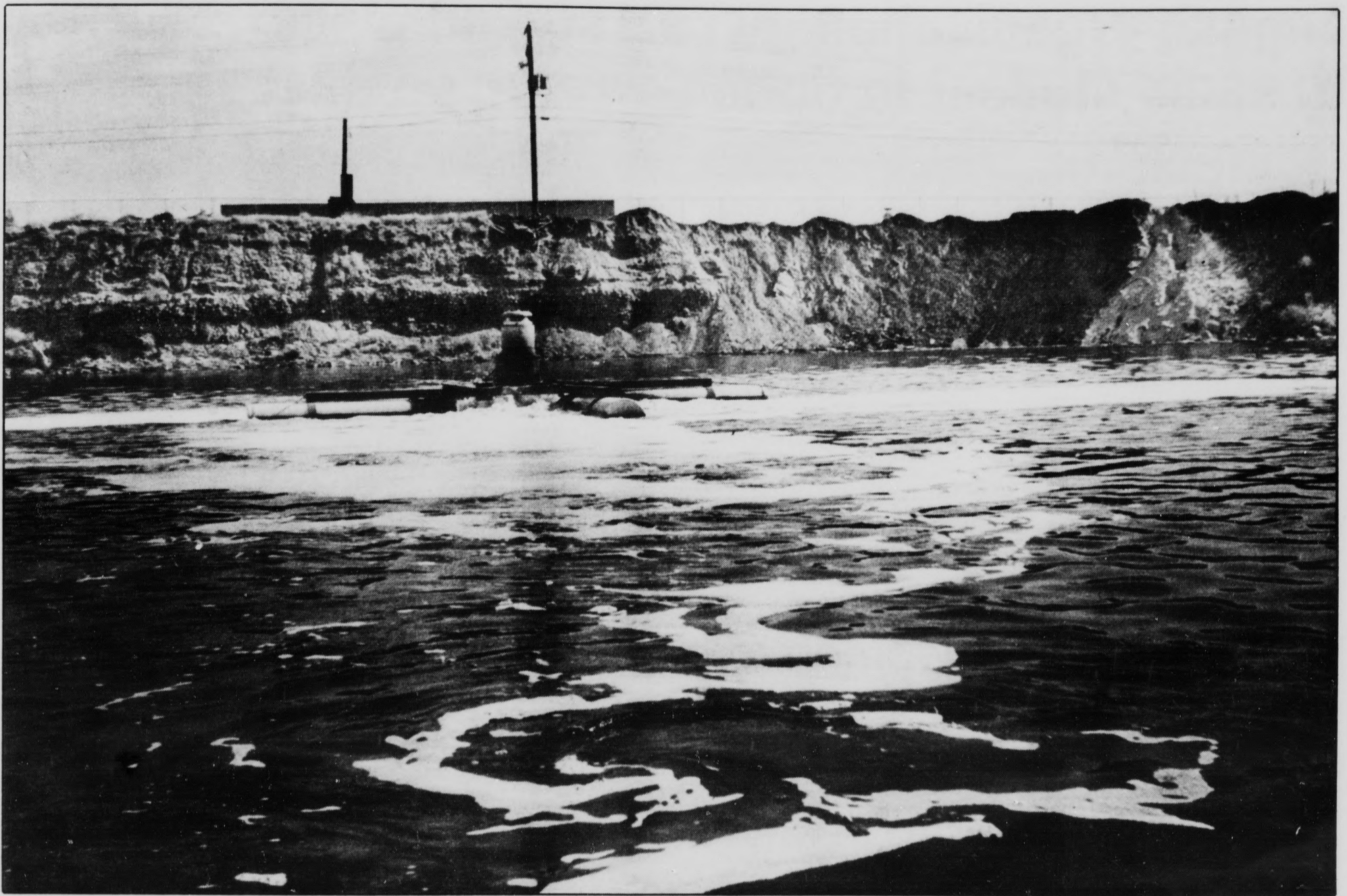
Does this look like a typical view of a lake? Take a second look. Floating on the surface of the water is one of three aerators that the owner of the landfill was ordered to install by the Arizona Department of Health Services. The machine pumps air into the water, encouraging algae growth. Ideally, the oxygen level will reach a point in which the algae will grow on its own.
