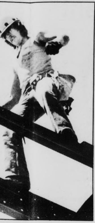
Worker for Eagle Steel Erectors Inc. works along two steel girders.
