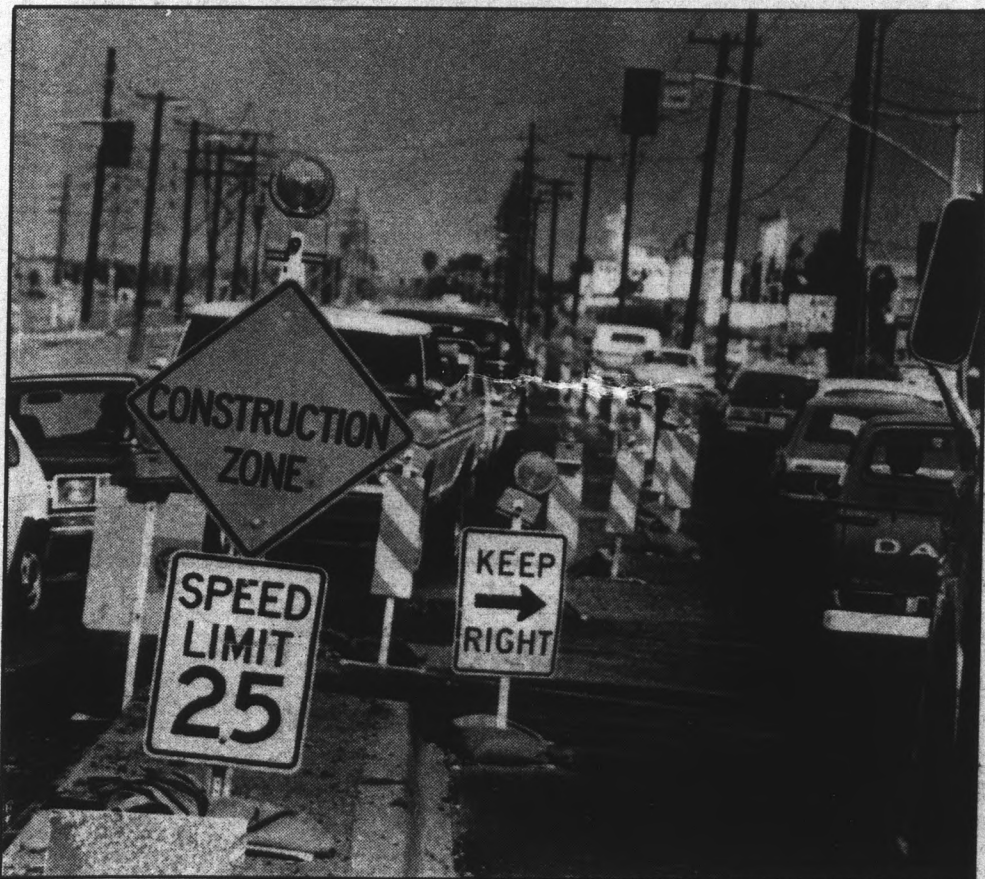
Drivers experiencing inconveniences from the ongoing construction on University Drive between Rural and McClintock Roads may be slightly consoled by the city's promise for a better street soon.
