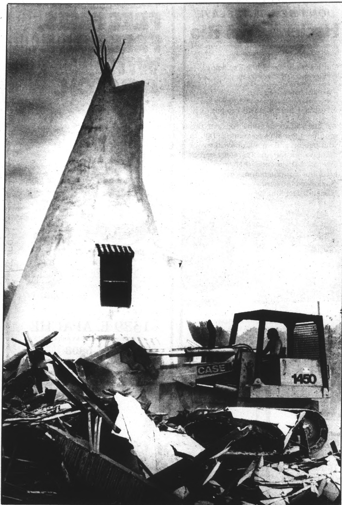
The last remaining teepee towers over a bulldozer clearing the remains of its neighbors.
