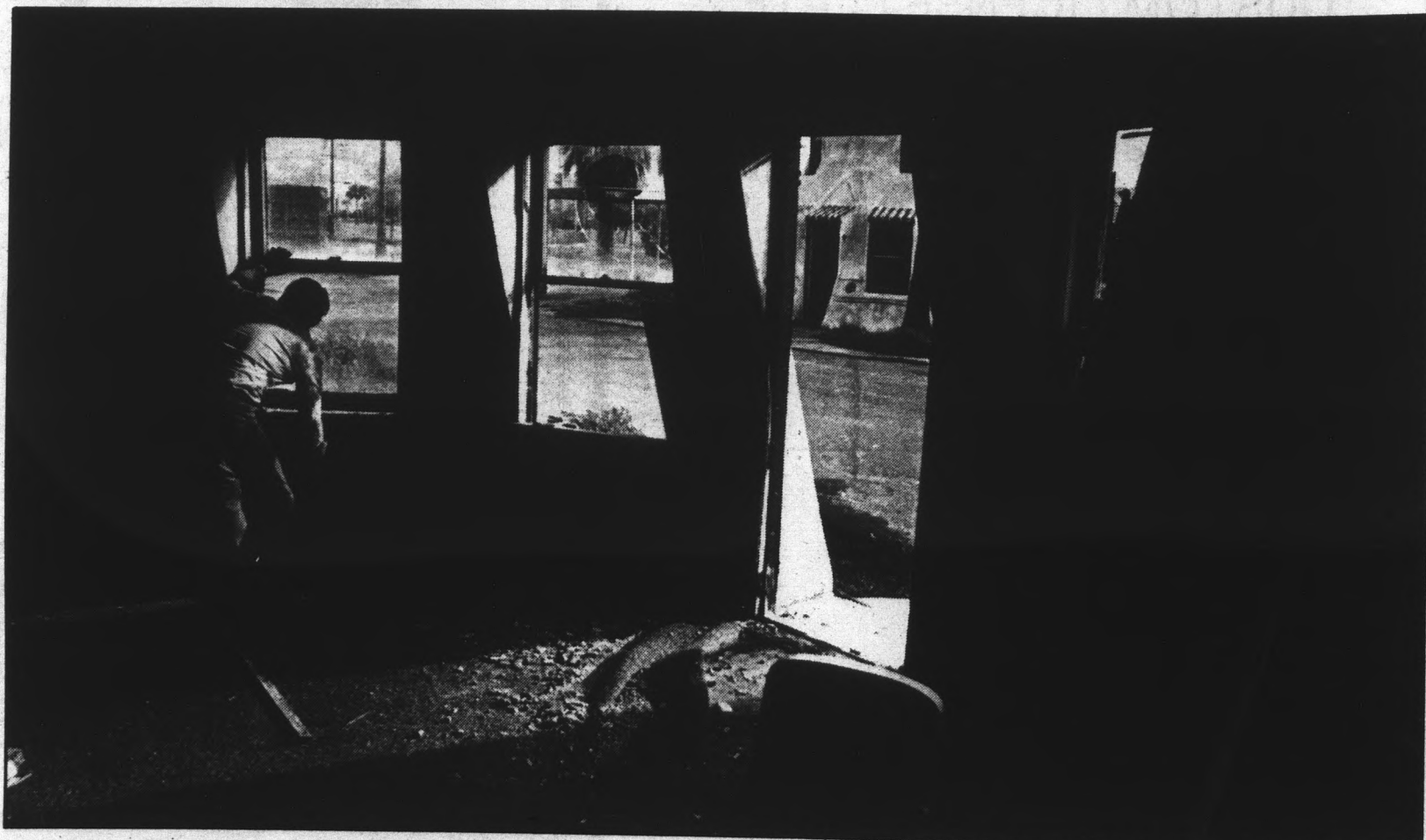
A member of the wrecking crew pries off a salvageable window.
