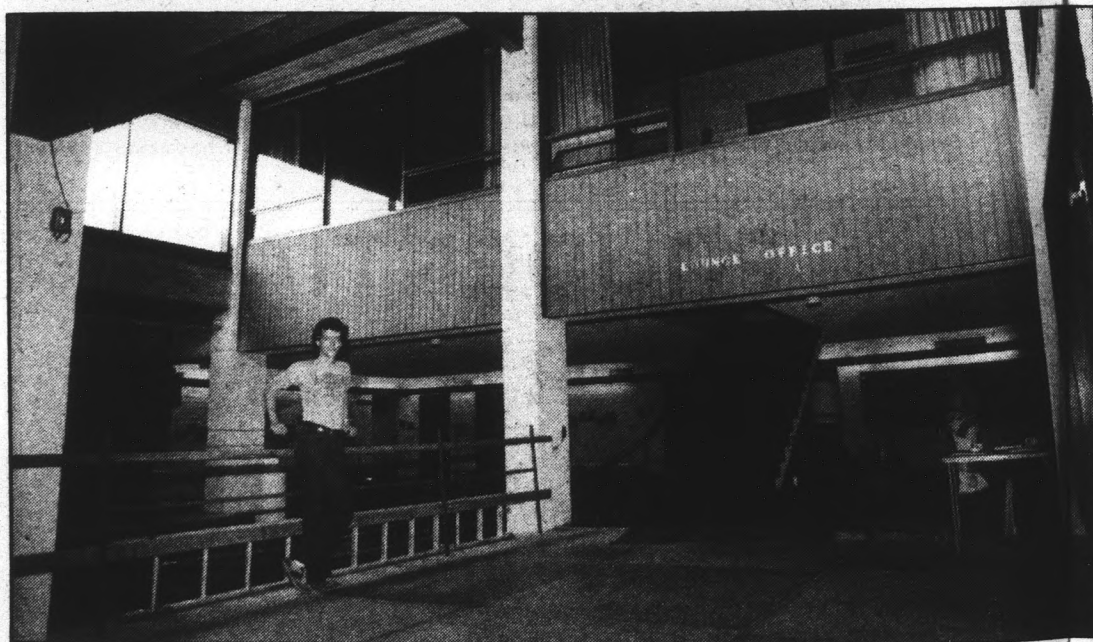
Steve Bachman, a senior mechanical engineering student and student council historian of the Newman Center, stands in the center's remodeled entryway.
