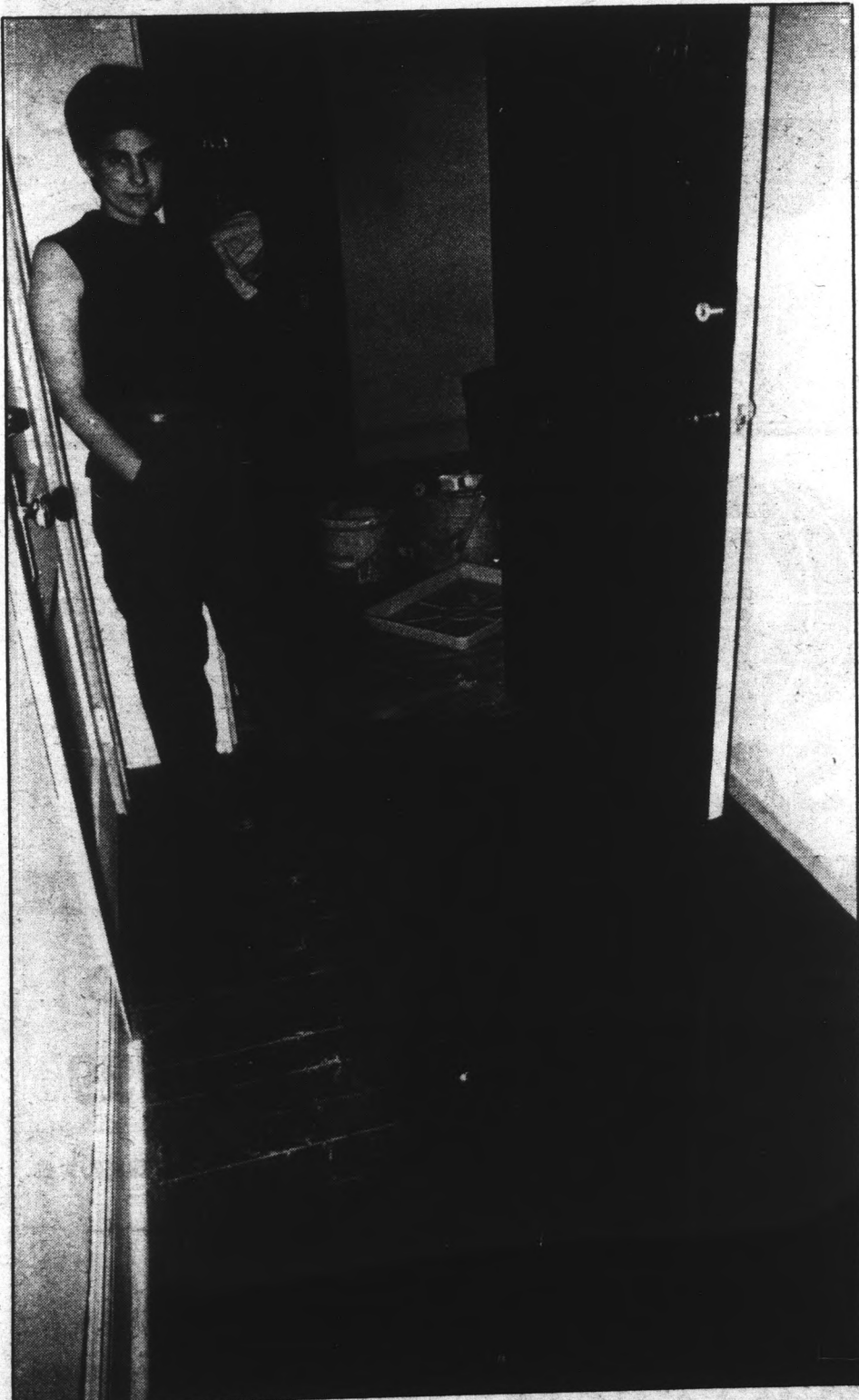
Lisa Sete, 23, a resident of Casa Loma, stands in the doorway of her third floor apartment. Sete claims there is water in the entry hall every time it rains. Right: The Casa Loma apartment building at Fourth Street and Mill Avenue.
