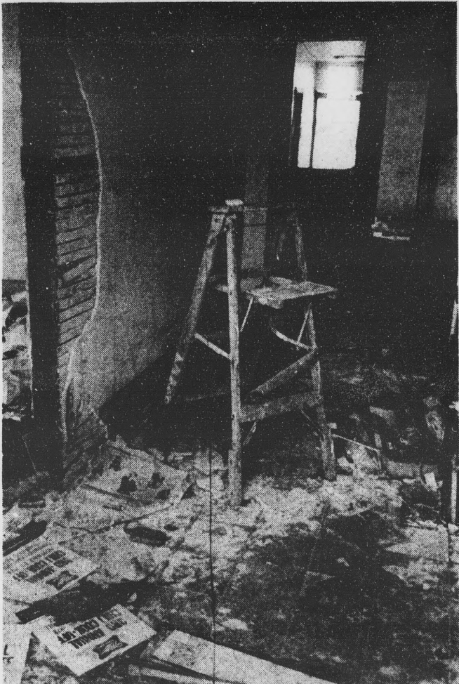
Turn-of-the-century house on Maple Street in Tempe is scheduled to be torn down for construction of a parking lot. [Photo by Dave Ryan]
