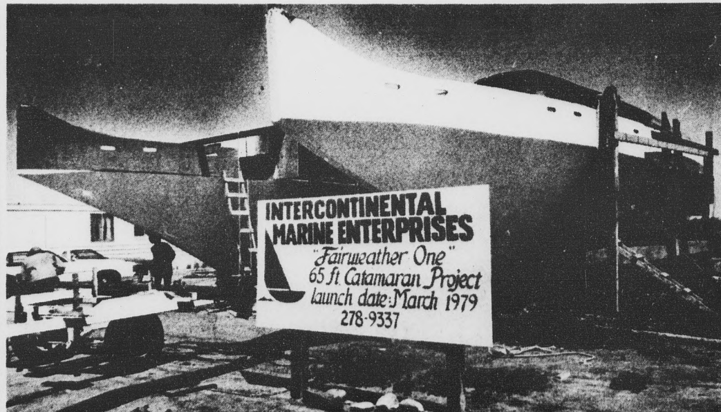
"Fairweather One," which was planned for completion in March, is now scheduled to be launched in May.
