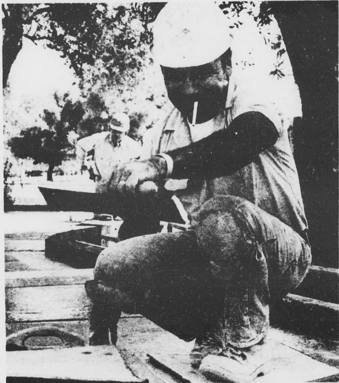
Henry Robertson is doing the trowel finish work for the sidewalk of the newly constructed office and classroom building. Construction of the new building will be finished within three weeks. [State Press photo by Matthew Liu]
