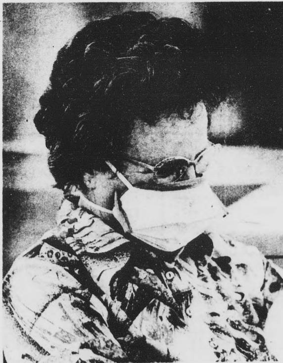
Helen Clark, a worker in the Moeur Building, is one of a number of people who have been wearing masks while cleaning out file cabinets. The mask protects them from asbestos particles they suspect to be harmful to their health. [State Press staff photo by Tony Corso]
