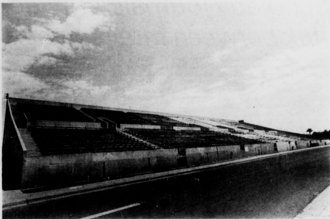
The final remains of Goodwin Stadium, the east stands, will be torn down soon, but the memories will linger on. [State Press staff photo by Mary Connell]
