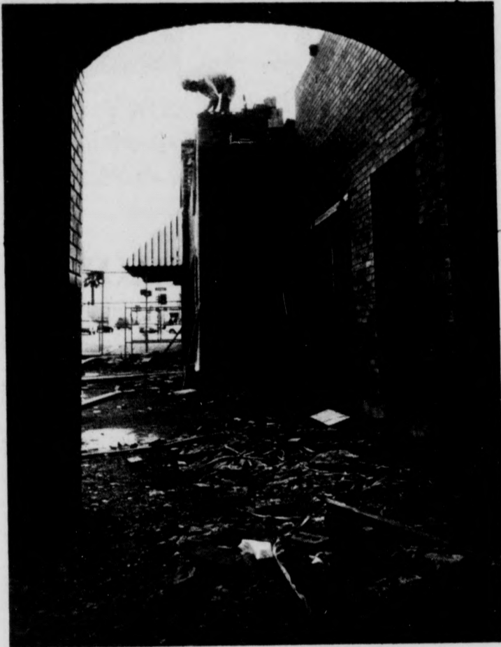
The arch of a bookstore under construction at the Mill Avenue Redevelopment Project frames bricklayer Victor Stewart. The first phase of the project is expected to be completed in three weeks. [State Press staff photo by Rhonda Prast]
