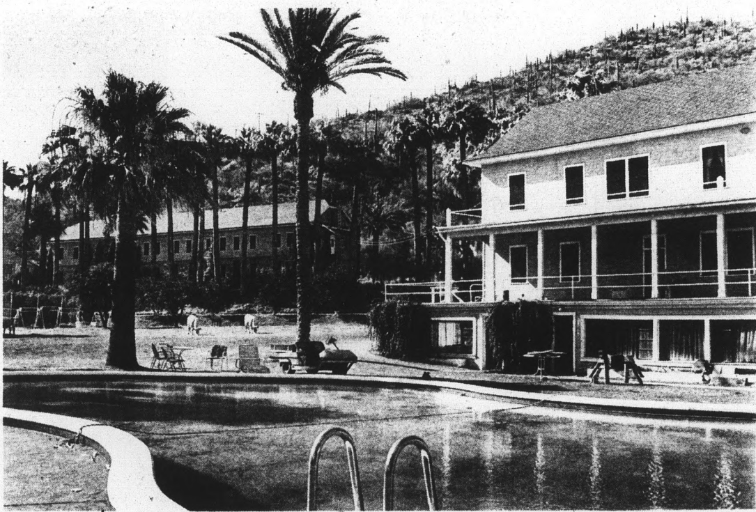
Castle Hot Springs, which was recently given to the ASU Foundation, is being readied to serve as a conference center. Remodeling is being done due to a fire which destroyed part of the resort in December. It will only be open to people participating in University-related seminars.
