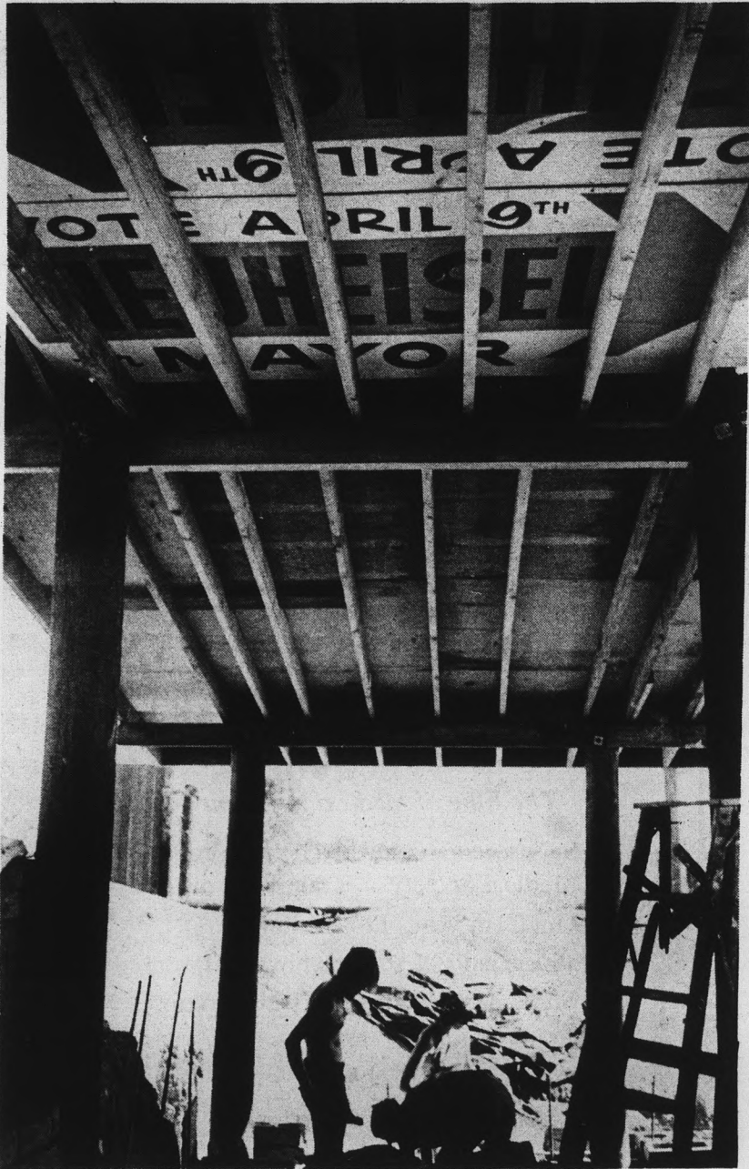
Architecture students are building a house entirely out of free materials. Part of the ceiling, above, is made of salvaged campaign billboards.
