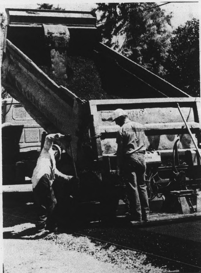
Pavers work on Forest Ave. mall.
