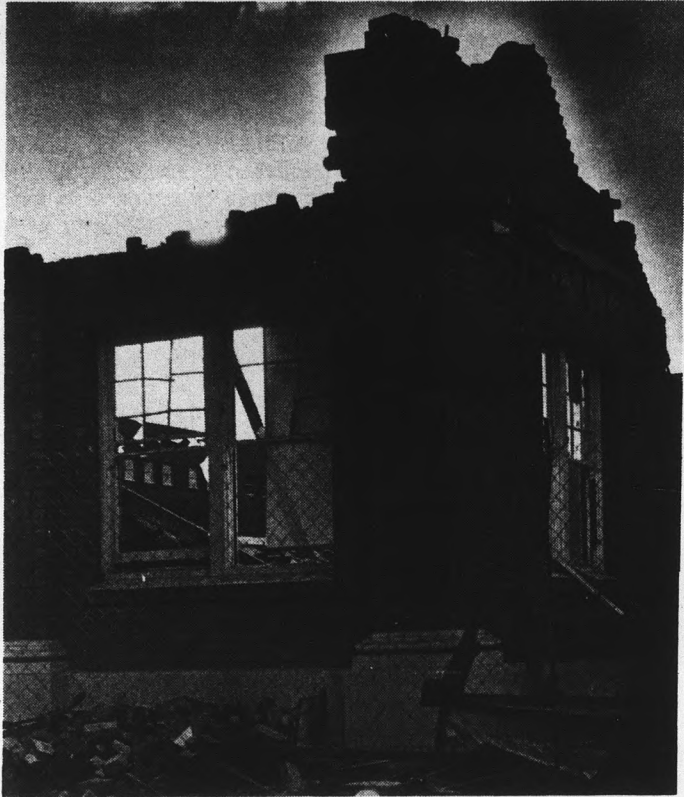
By today the remnants of 58-year-old South Hall will have been knocked down and only the rubble will remain to be hauled off. The University decided the cost of prolonging the usefulness of the termite-infested hall was too great.
