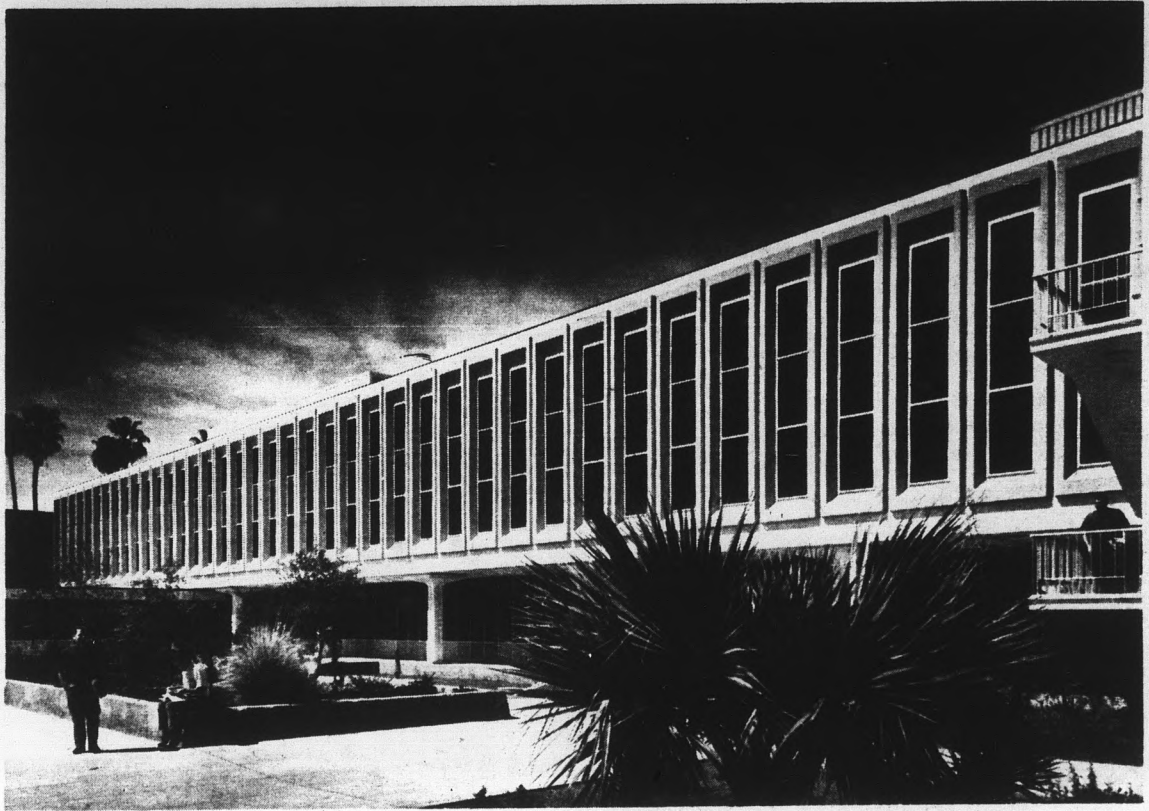
One of several wings of ASU's Engineering Center
