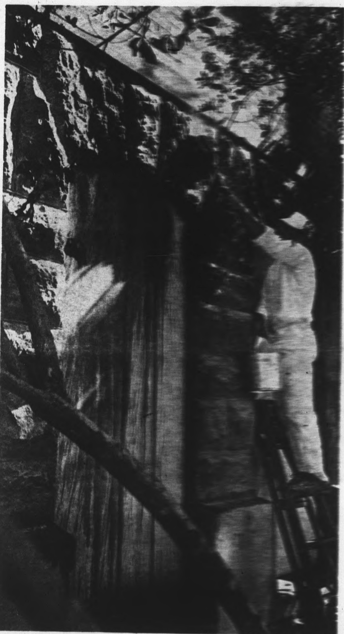
Old Main damage repaired
