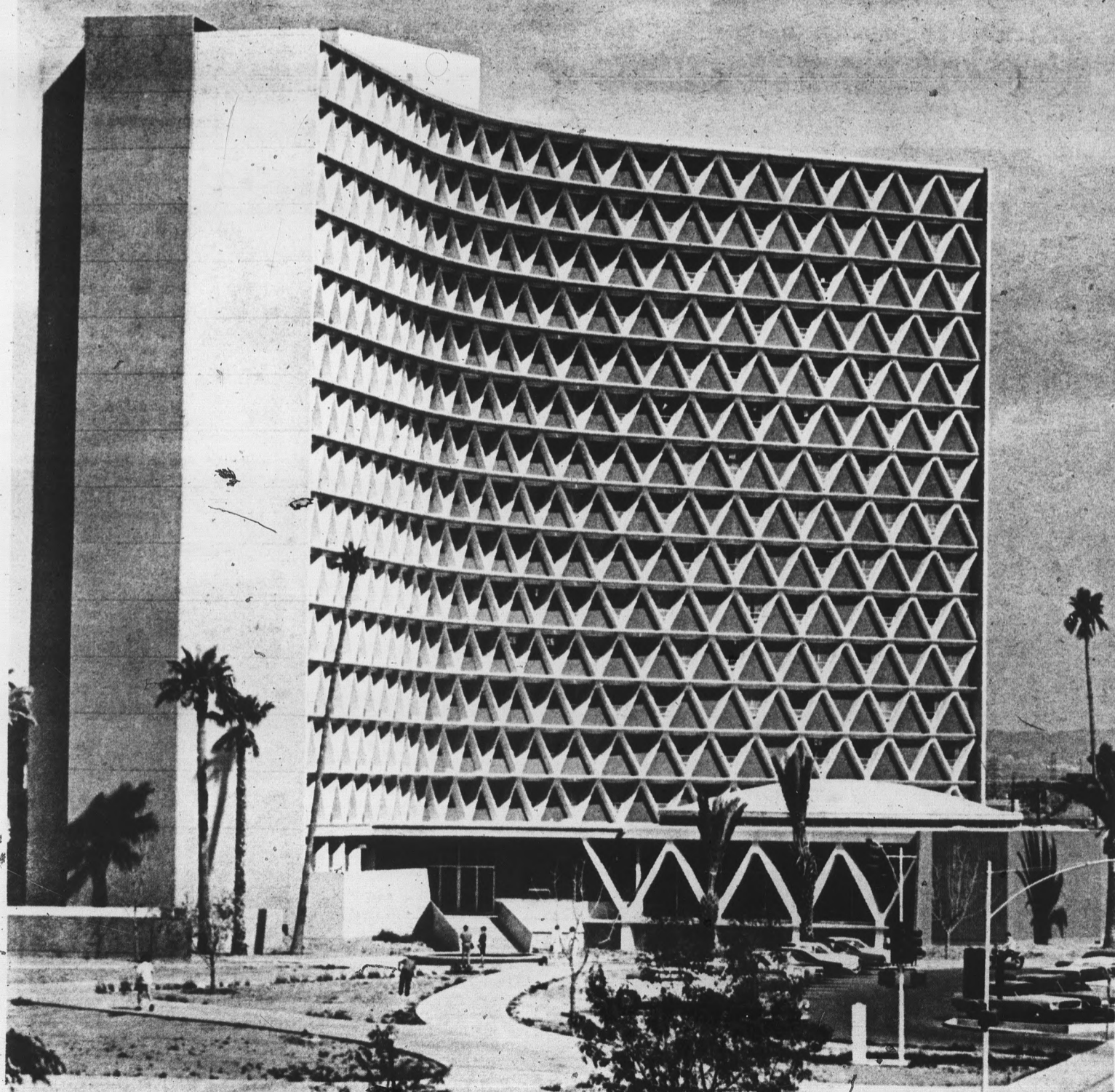
Manzanita Hall women's dormitory — tallest building on the Campus
