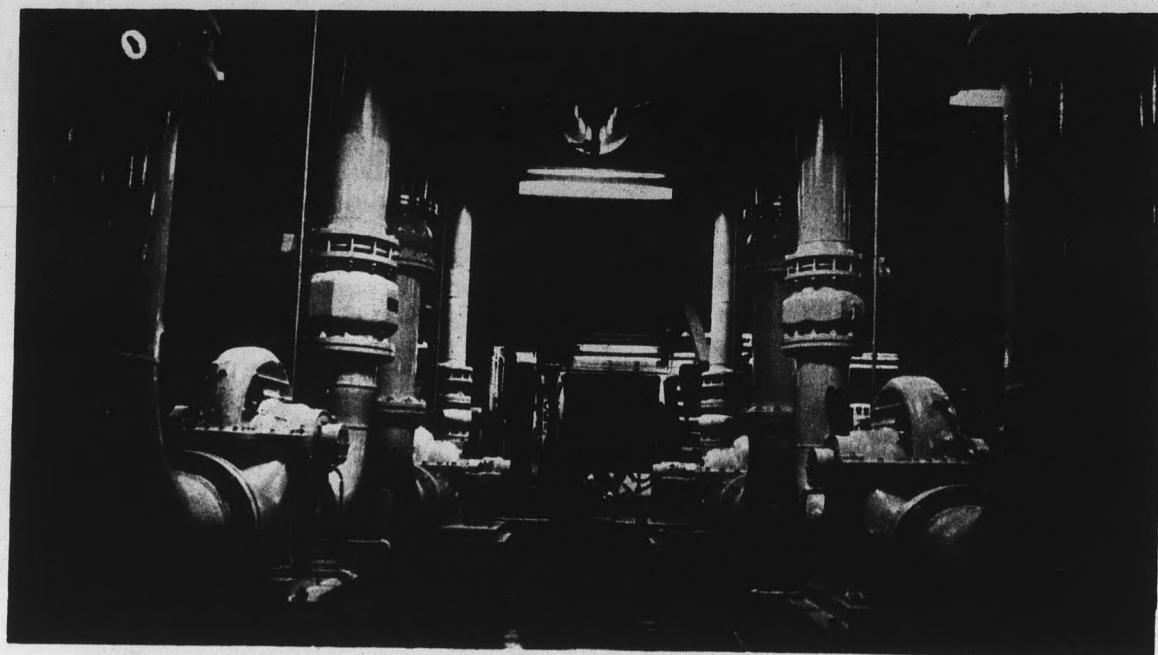
Huge air conditioning units will be shown tomorrow at Physical Plant open house.
