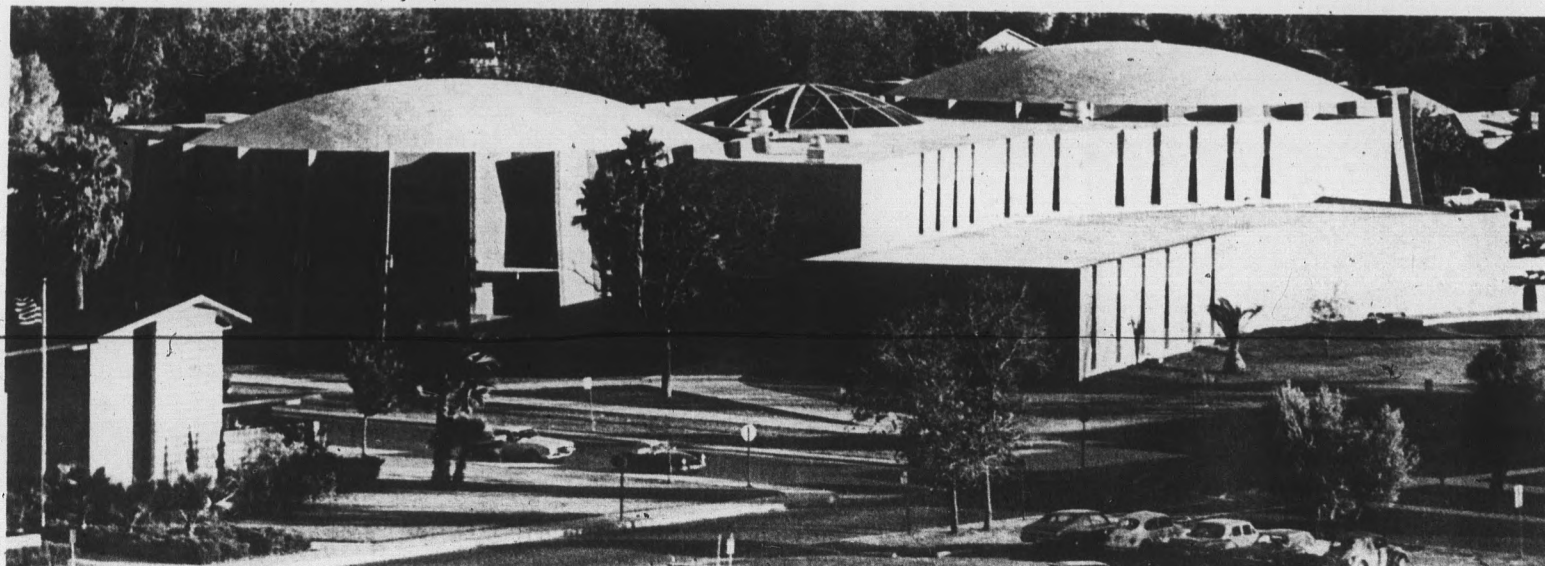
LAW COLLEGE — ASU's current class of prospective lawyers is headquartered in this modern structure.
