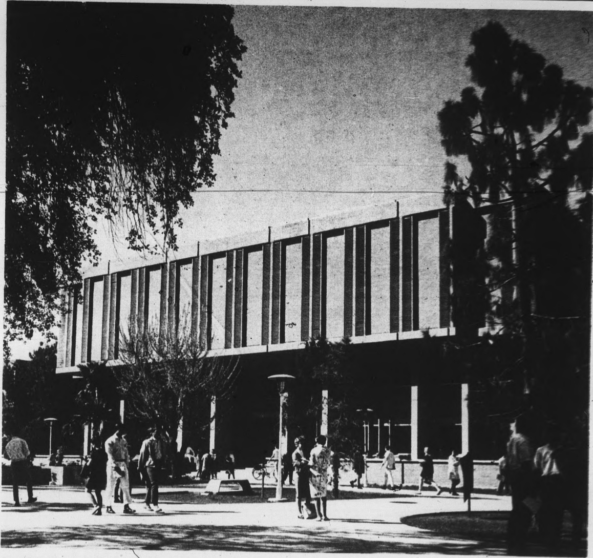
NURSING CENTER — Housed in this structure are College of Nursing and Graduate School of Social Service Administration.
