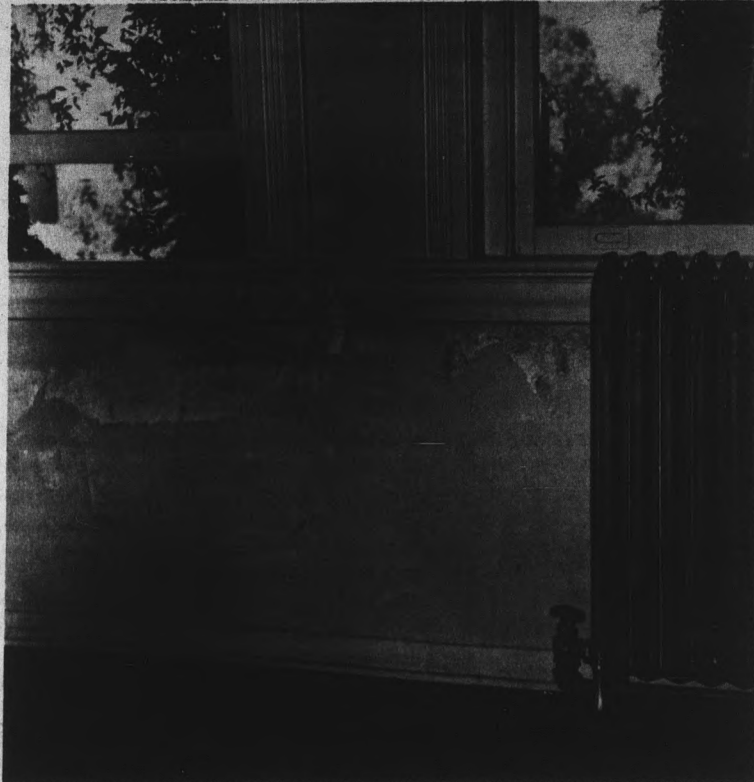
A BIT OF RUSTIC ARIZONA — Old fashioned iron steam radiators have been used in combination with open windows to provide rooms' occupants with heating and cooling. Next semester the building will be shut down so a more modern system can be installed.
