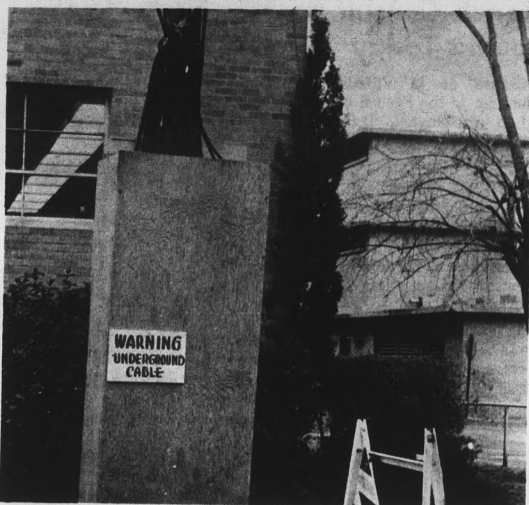
PROTECTIVE SHIELD — This wooden structure is evidently designed to protect students from any dangerous electrical wiring temporarily attached to the telephone pole. But the sign warns of underground cables against which there is no protection. Hmm . . . a little incongruity there.
