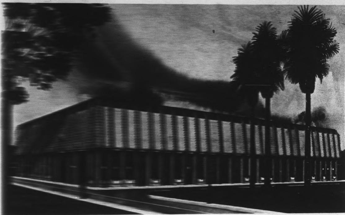
REMODELED HEATING AND COOLING PLANT... Cost will exceed $1.5 million.
