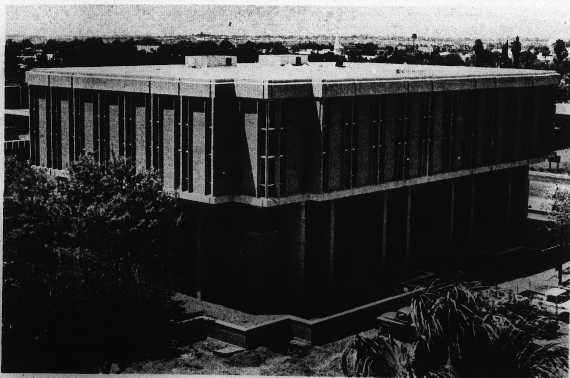
READY FOR FALL — Four stories tall, the University's new College of Nursing building is nearly completed. The new facilities are eagerly awaited.
