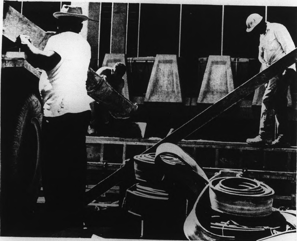
CEMENT, NOT DUST — Walkways of cement will soon skirt the new library instead of the thick dust that now surrounds most of the construction.
