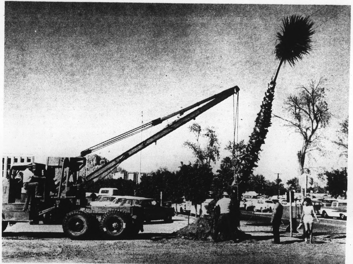
GOING DOWN — Workers plant palm trees at the east end of the engineering building. Sidewalks in front of the building were poured yesterday as construction comes to a close.
